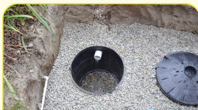
Rain Water Harvesting Pits
